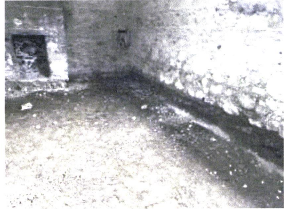
Replacement ground floor with a new insulated sla
