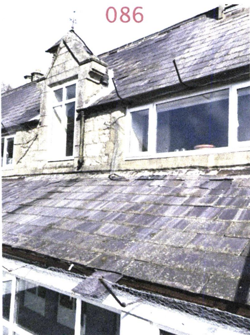
Roofs to Club Room Buildings - Cupolas in a state of total disrepair.
