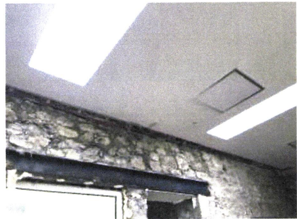
Treat existing steelwork with corrosion protection.
