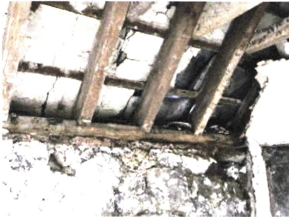
Replacement wall plates in accordance with timber conservation specialists report
