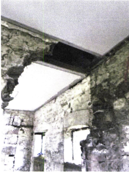
Install replacement head with PC lintel and reconstruct masonry wall over.
