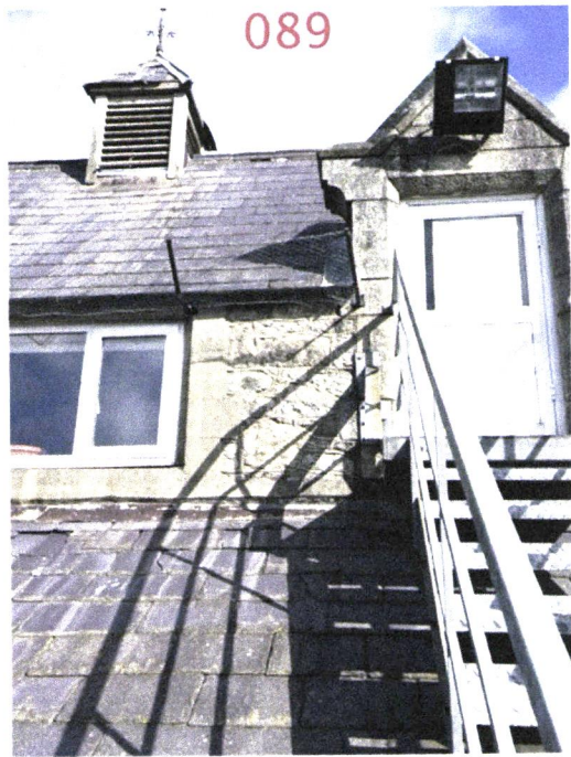
Roofs to Club Room Buildings - Cupolas in a state of total disrepair.
